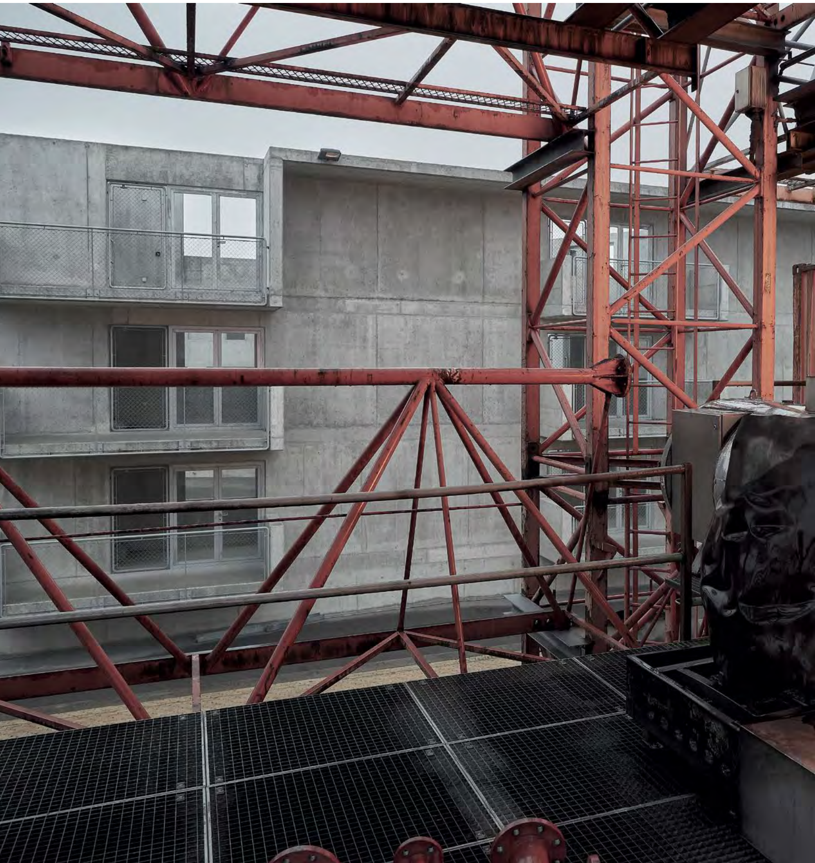
In the foreground: the industrial fire extinguishing practice facility. Here, several teams can train to master eleven different fire sources that are centrally remote-controlled by hand. In the background: the façades of the "row houses."
